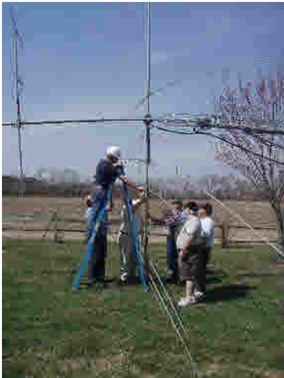
An Antenna Party at Dick's -W3GNQ house to repair damage to his Force 12 40M Beam from the winter storms.
